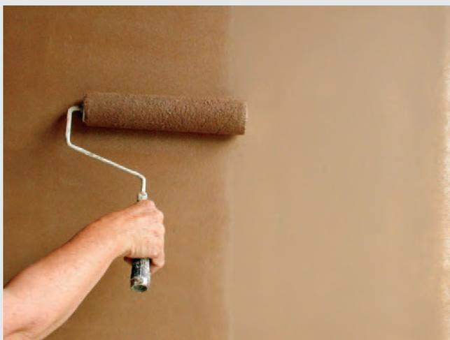
3. The final topcoat may be done two ways. Apply directly with the larger brush in a crisscross manner or use the roller to apply an area of paint about a metre square and use a dry brush to create the criss-cross effect. Do some test boards first and use whichever technique you find easiest. Make sure you use the same method for any other areas so that the finish looks consistent.
