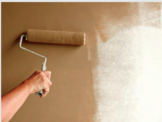
2. Apply a coat of Resene Axis using the same method as above. Take the roller as close as you can to the edge of the wall then finish by laying off in one direction.
