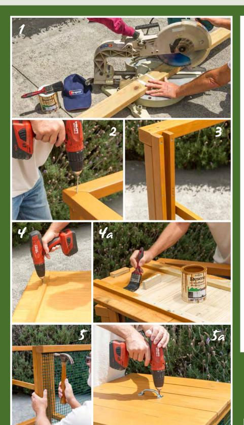
**Step 1:** Using the drop saw, cut the framing and corner posts to the lengths noted opposite. Mitre two ends of two pieces of the 650mm, and one end of the other four. Screw them together to form the top and bottom frames.
