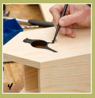
Draw a bird shape around the hole with the foot ending on the peg and paint with Resene Black. Or you can jigsaw the shape instead. Paint the peg and insert it. Paint the roof, using a Resene testpot (which is fine for outdoor use). We used Resene Clockwork Orange.
