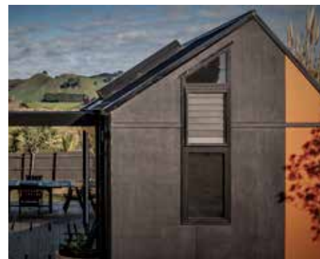
left: Cladding in Resene Sonyx 101 CoolColour tinted to Resene All Black. Accent in Resene Ayers Rock. Design by Tohu Workshop of Architecture, www.tohuarchitecture.co.nz. Build and painting by Mustard Builders, www.mustardbuilders.co.nz. Image by Sharni Dysart, www.instagram.com/sharni_dysart_photographer.
